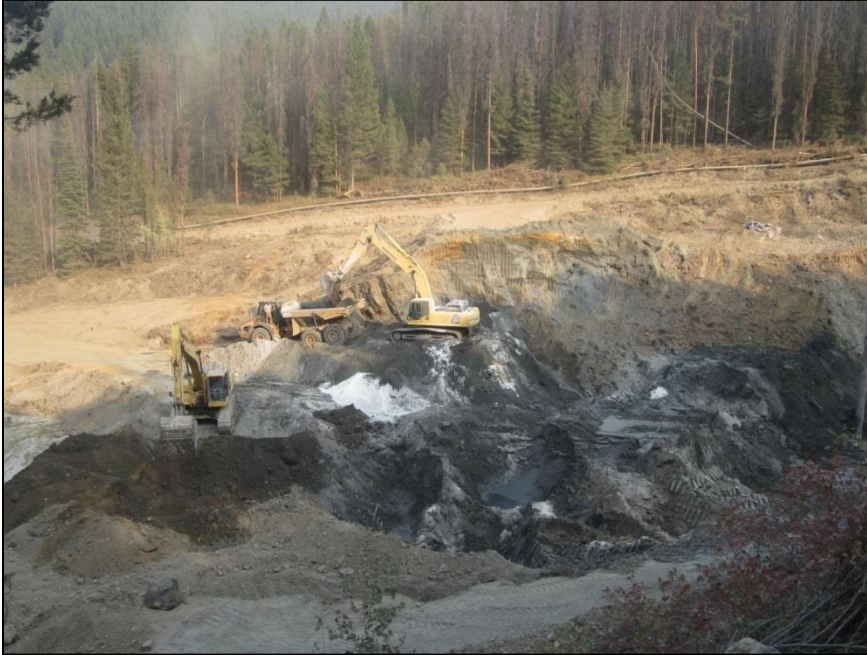
Photo: Excavation of tailings at the Forest Rose Project site.
