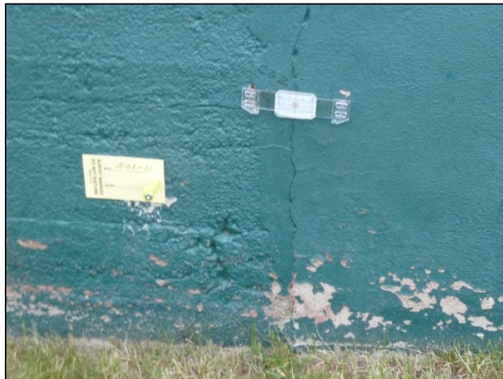
Photo: One of several crack monitors installed on the foundations of homes in Red Lodge where subsidence concerns have been expressed.
