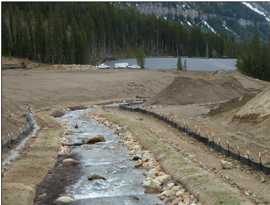
Photo: Recently reconstructed stream channel (Soda Butte Creek) through the project area, with the installation of the top geonet layer on repository occurring in the background during the OSMRE site-visit on June 19, 2014.
