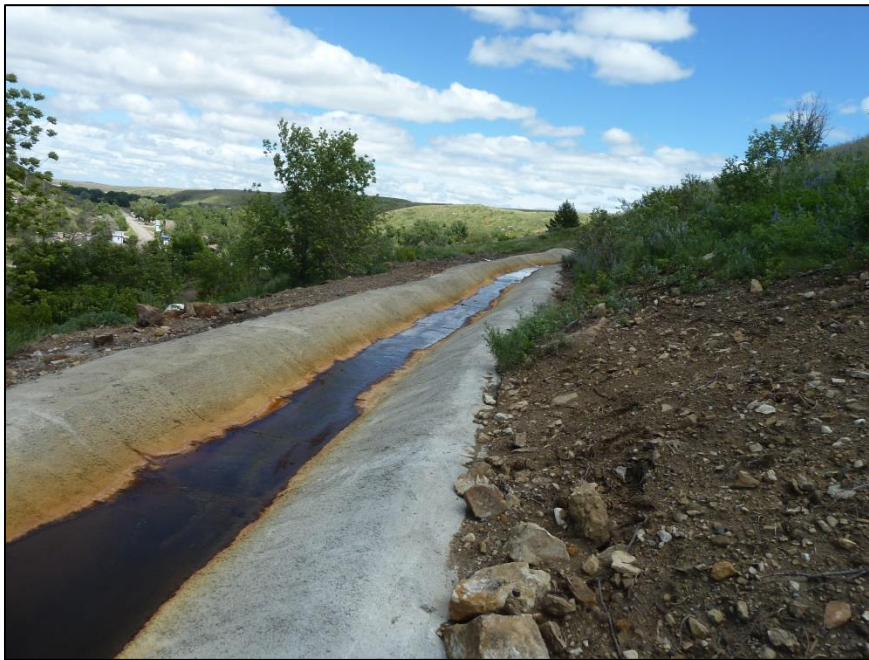
Photo: Lined ditch constructed above the town of Sand Coulee, photo taken during OSMRE site visit on June 17, 2014.
